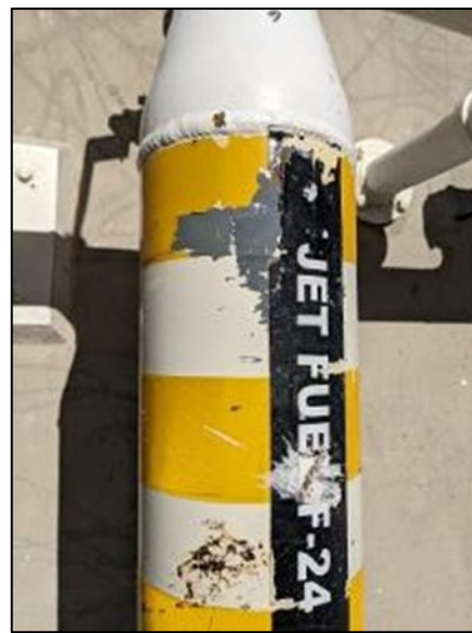
Photos 4 and 5 Raven Caused Corrosion of Facilities at SELF
