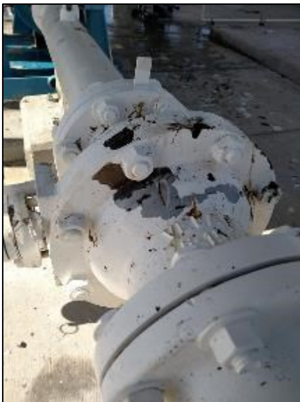
Photos 4 and 5 Raven Caused Corrosion of Facilities at SELF
